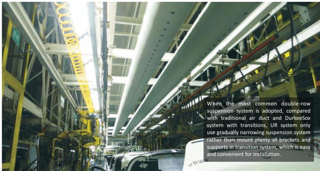
When the most common double-row suspension system is adopted, compared with traditional air duct and DurkeeSox system with transitions, UR system only use gradually narrowing suspension system rather than mount plenty of brackets and supports in transition system, which is easy and convenient for installation.
