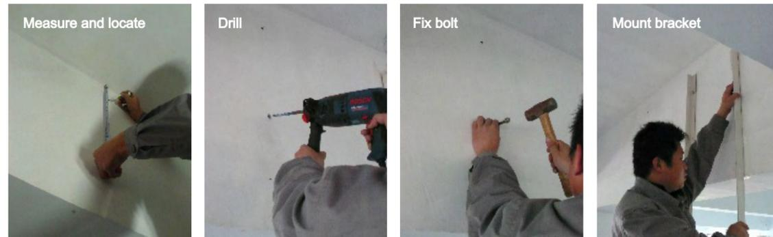
Determine the spacing and height of tension cable according to height and diameter of each metal duct outlet. Determination of bracket spacing requires that the front and the rear brackets of the same DurkeeSox system should be mounted parallel and symmetrically without any deflection.
