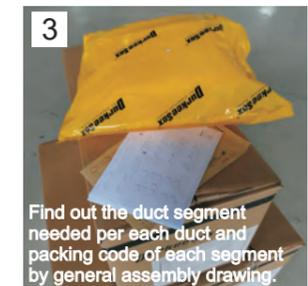
Each duct segment of standard length has been put into a plastic bag containing a product installation and assembly drawing, which has the information on the corresponding duct diameter, length, orifices orientation and the specific position for installation. Furthermore, there is a label at the inlet or near the zip of each duct segment, The label indicates the diameter, length, duct code and segment number of the duct.
