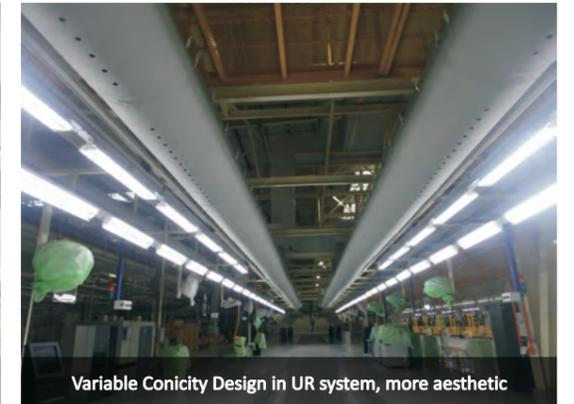
Variable Conicity Design in UR system, more aesthetic
