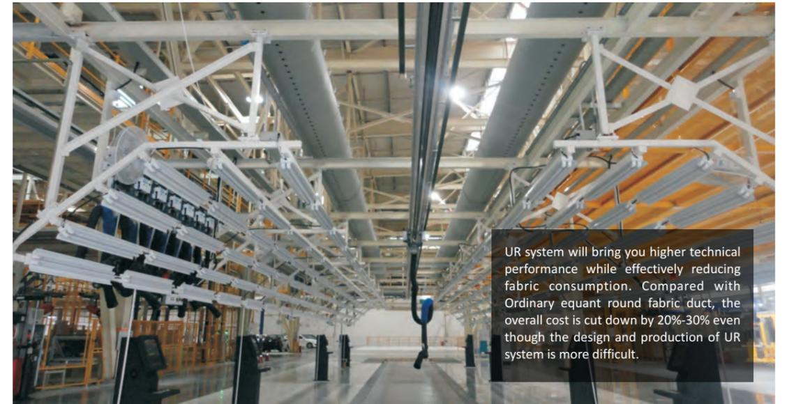
UR system will bring you higher technical performance while effectively reducing fabric consumption. Compared with Ordinary equant round fabric duct, the overall cost is cut down by 20%-30% even though the design and production of UR system is more difficult.
