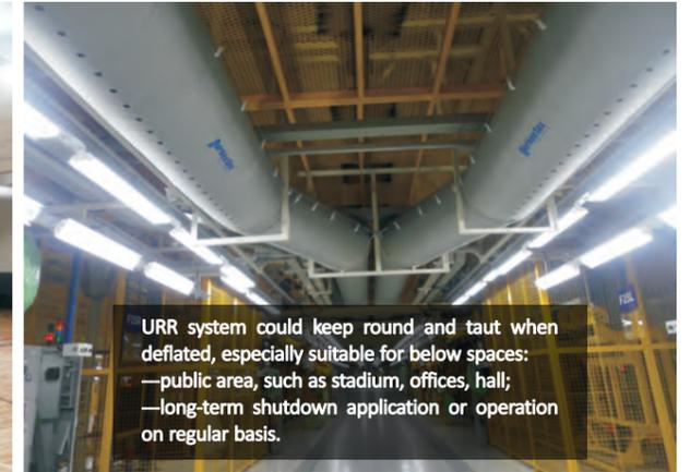
URR system could keep round and taut when deflated, especially suitable for below spaces:
