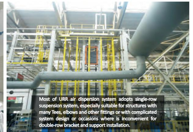
Most of URR air dispersion system adopts single-row suspension system, especially suitable for structures with many Tees, elbows and other fittings or with complicated system design or occasions where is inconvenient for double-row bracket and support installation.
